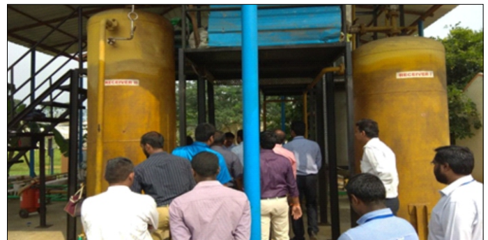
Industrial visit to 'CNG -Bio Plant' at Mahindra World City
